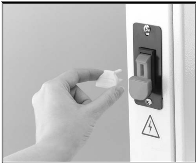
Figure 5. Remove safety key when not in use.
